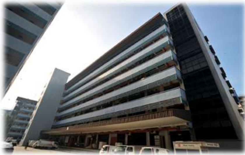
Toa Payoh North 1 Cluster before redevelopment
