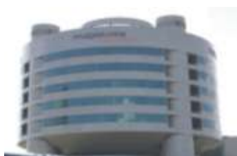
Business Park Buildings
